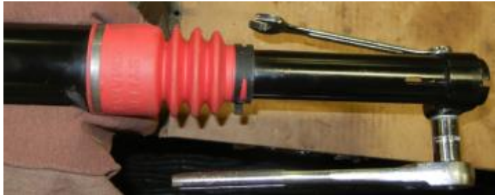
Figure 1: Bolt & Nut Removal
