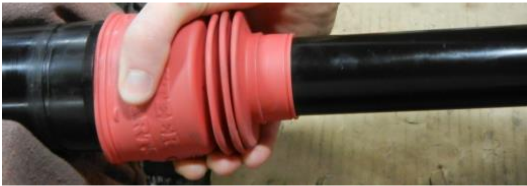
Figure 6: Bellow Seal Removal
